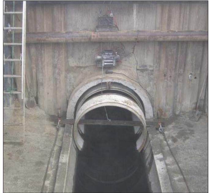
6. Immediately upon completing installation of the pipe it should be anchored to prevent movement. This is accomplished by pulling back on the safety cable into the pit and securing but not moving the installed pipe string. Block the downstream and upstream ends of the pipe ends with wood wedges. Air bags may be used on a temporary basis until the wood wedges are securely in place. NOTE: At no time after installation of the liner pipe in live flow shall the liner pipe be left unrestrained.
