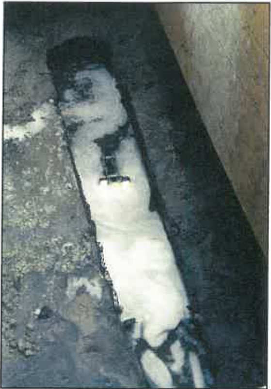
A track-mounted video inspection camera records the condition of the sewer line.
