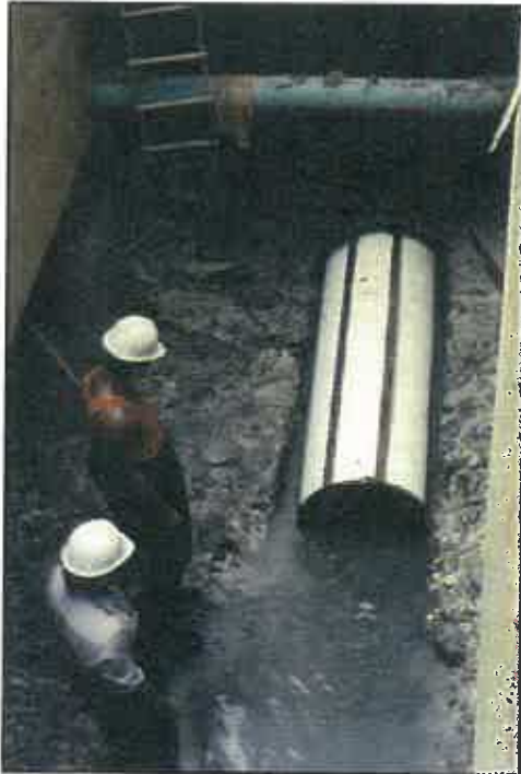
Boyer workmen watch as a mandrel begins a test run through the cleaned sewer.
