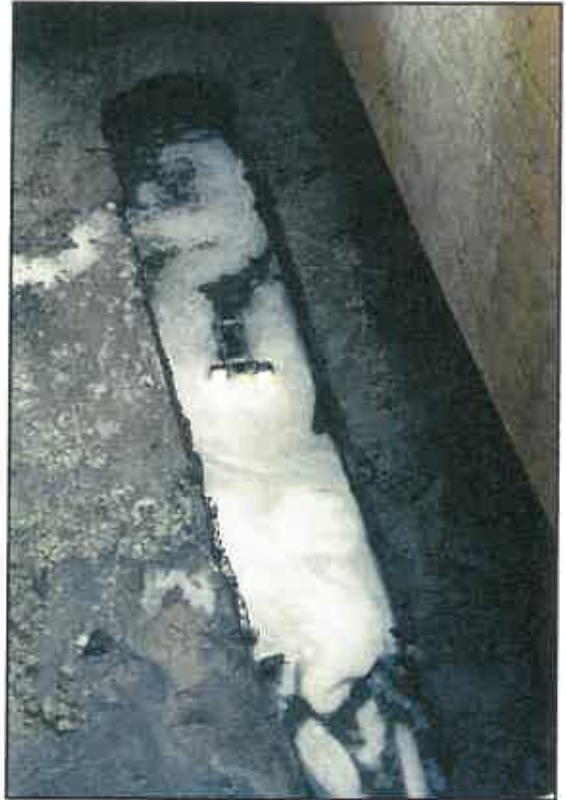
A track-mounted video inspection camera records the condition of the sewer line.
