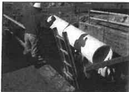
Slipline lowered into shored insertion pit.
