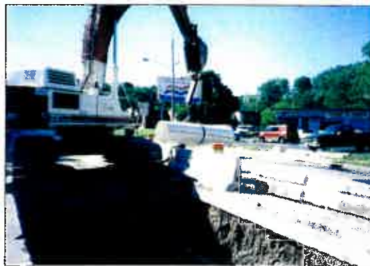
Marra Construction crews lower a 15-ft section of Lamson Vylon slipliner into the insertion pit.
