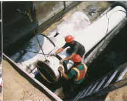
Metra Industries/Spiniello used Lamson Vylon PVC Slipliner to restore 2,400 ft of 36-in. ID concrete pipe in Ocean County, N.J.
