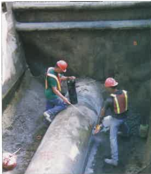
Metra Industries/Spiniello used Lamson Vylon PVC Slipliner to restore 2,400 ft of 36-in. ID concrete pipe in Ocean County, N.J.
