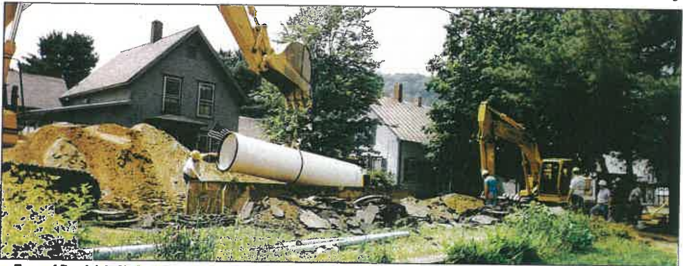
Town of Randolph, VT installs new stormwater system in response to combined sewer overflow (CSO) control policy.
