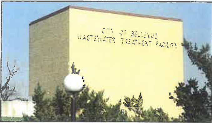
Wastewater Treatment Facility
